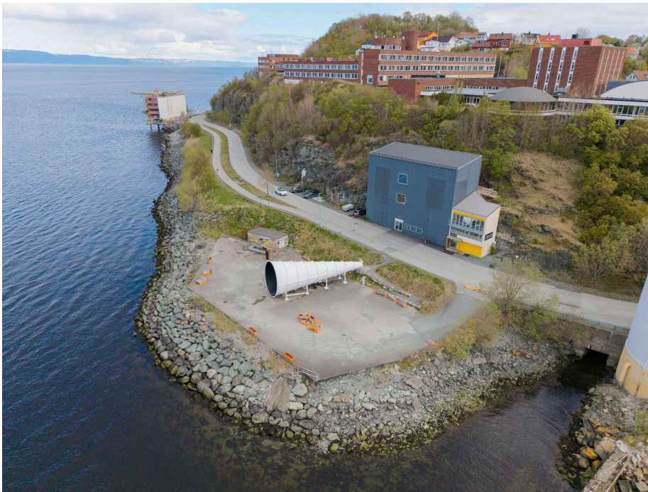
Photo by John Arne Hansen Tømmervold, May 2026 showing the intervention area. Source: Trondheim municipality
