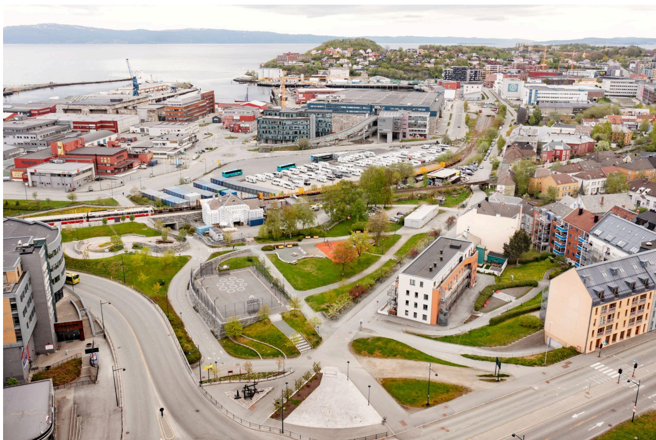
Photo by Glen Musk, May 2022 showing the intervention area before transformation. Source: Trondheim municipality
